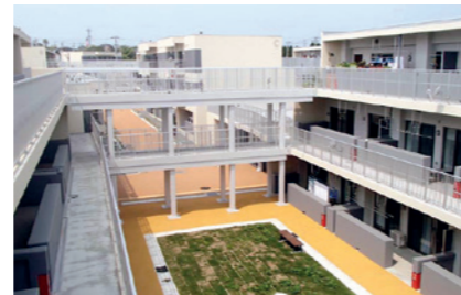
Photo: Disaster public housing in the Shobutahama district of Shichigahama Town
