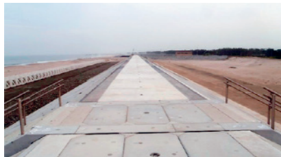
Photo: Arahama Seawall (Watari Town)
