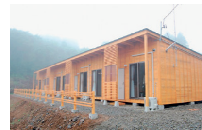
Photo: Temporary housing made with local lumber (Minamisanriku Town)
