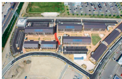
Photo: Solar power system providing power for disaster public housing (Ishinomaki City)
