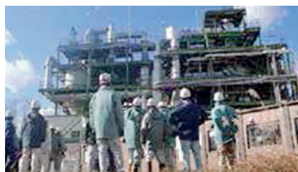
Photo: Restoration of sludge incineration facility completed at Senen Purification Plant
