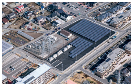
Photo: Ishinomaki Hebata Solar Power Plant (Ishinomaki City)
