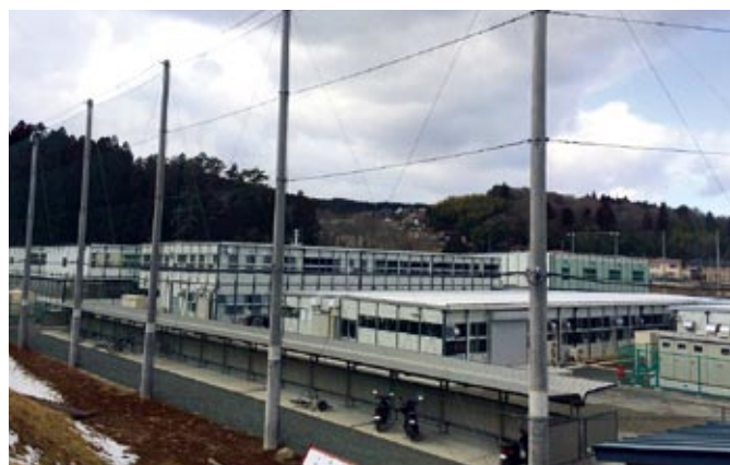
Temporary school building of Kesenuma Koyo High School (Kesenuma City)
