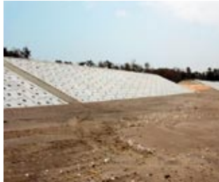
Photo: Restored coastal levee (Shichigahama Town)
