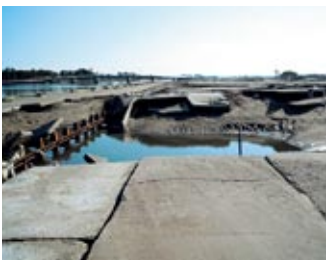
Photo: Damaged Yuriage Port (Natori City)
